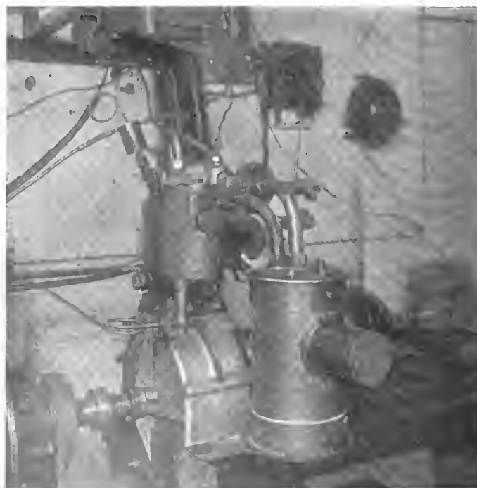
CARBURETING CHAMBER AND CONNECTIONS.
